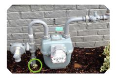
The yellow tracer wire needs to remain in place. This wire is used by the gas company to locate underground pipes.
