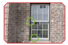
Check caulk joint between window and bricks around the entire periphery of window. There should be no gaps. All windows caulk joints on the exterior of the house should be examined once a year to ensure that there are no caulk breaks/gaps from the windows to the brick. A good caulk joint is necessary to provide a tight water and air seal to prevent water leaks on the inside of the house and to maximize heat and AC efficiency.
