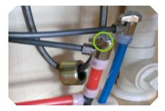
Each toilet has a shutoff on the water supply line located under the tank. The small valve can be rotated 90-degrees to stop the water flow to the tank. Hot and cold water shut offs for each sink are on the water lines under the sink.
