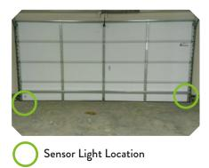
Your garage door is equipped with two sensors at the bottom right and left hand corners for safety; these sensors detect objects while the garage door is in motion. Once an object has crossed the sensor beam while door is in motion the garage door will go back up to keep from closing on object.
