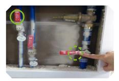
The main water manifold is usually located in the wall in the garage and has the control valves to shut off water flow to the entire house and to outside hose bibs. It is recommended to winterize your hose bibs during freezing temperatures. Once you have shut-off the water to the hose bibs go outside and drain any excess water out and then turn the hose bib to the OFF position. (In case of an emergency or for conducting any plumbing repairs)
