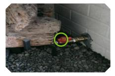
Make sure the gas valve located to the right of the fireplace logs is in ON position. The red valve should be in line with the gas line.
