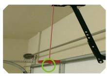
Your Garage door is equipped with an emergency pull cord in case of power outages. This allows you to operate the garage door manually. This pull cord is red in color and has a handle. The pull cord is located on the top rail system hanging down.
