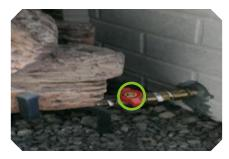
The fireplace can be turned off by rotating the ON/OFF/PILOT knob to off position. This will extinguish the pilot light. You can also turn the gas valve to the off position to stop the flow of gas to the log unit.
